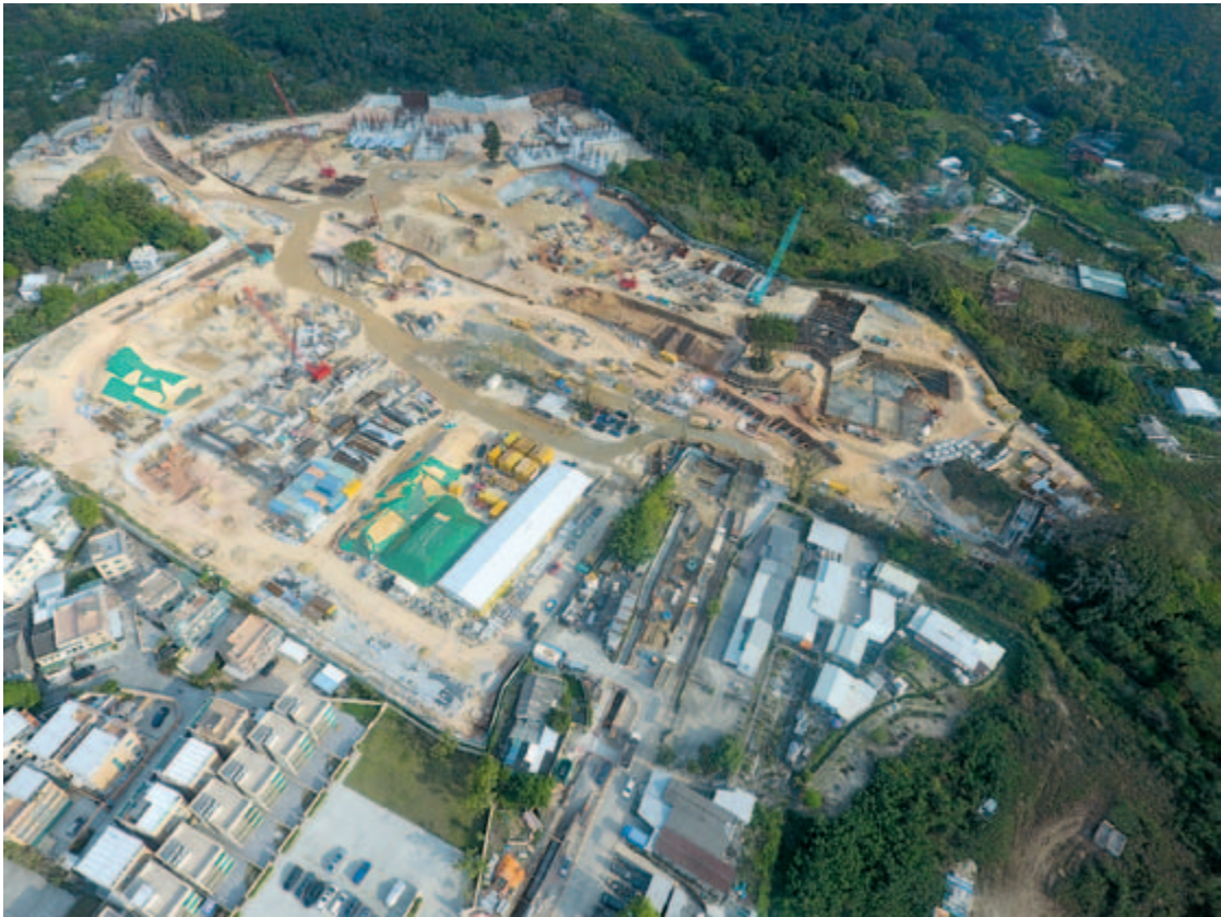
Aerial view of Queen's Hill Project
