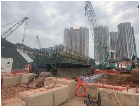
Sludge dewatering system was installed to the construction site
